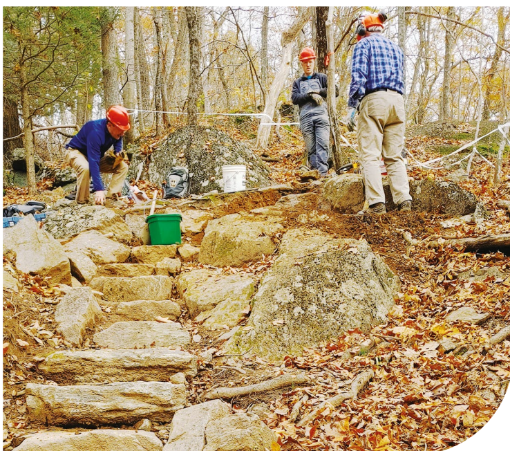
Steep Rockers laying 20 steps on Meeker Trail, Macricostas Preserve
