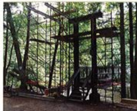
Tower structure repair/replacement at the Hauser Bridge
