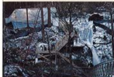
New stairway to replace access ramp at the Reich Bridge
