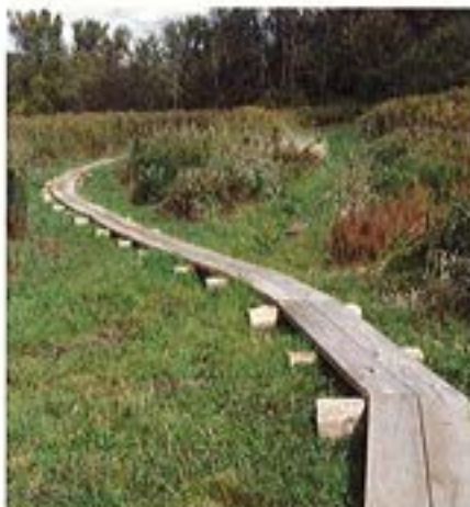
New boardwalk meandering through the meadow at Macricostas Preserve
