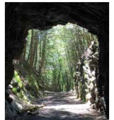
Railroad Tunnel at Steep Rock Preserve
