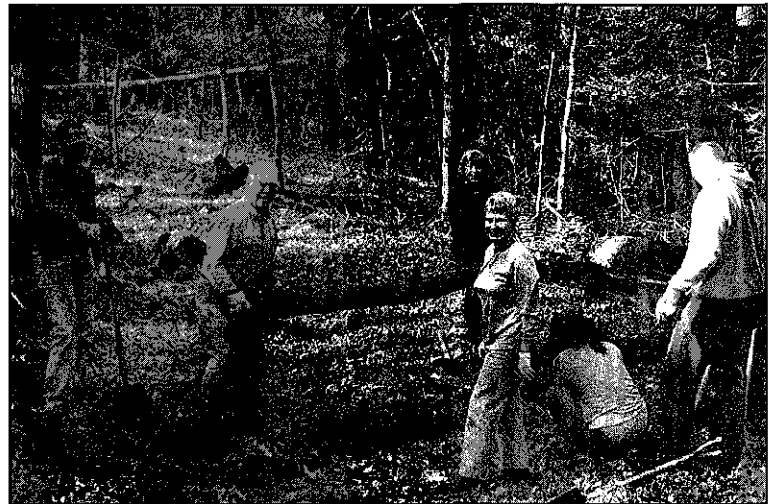
From left, Trustees Jane Conn, Chick Treadway, Natalie Dyer and Kirsten Peckerman and volunteers Cynthia Carter and Steve Paggioli building and installing a waterbar. This fall workday in Hidden Valley focused on directing water flow from the hillside off the trail.
