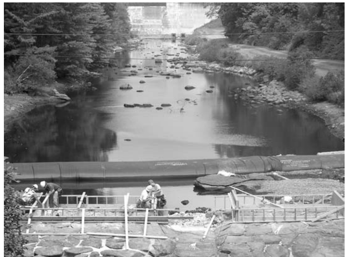
Construction at Peter's Dam, below the Shepaug Reservoir
